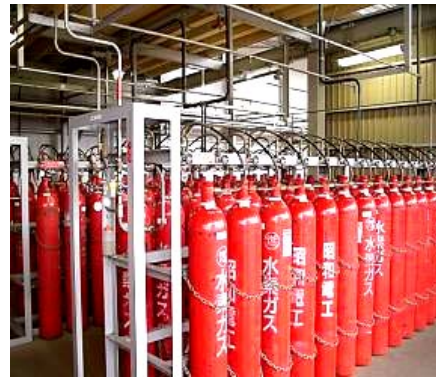
Photo 5: An example of marking on hydrogen gas containers
