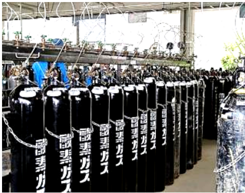
Photo 4: An example of marking on oxygen gas containers
