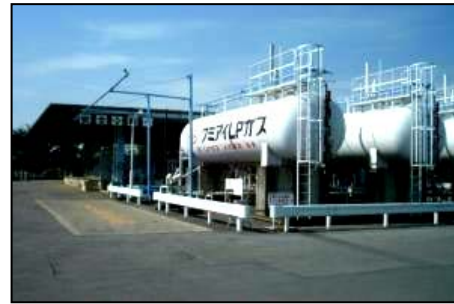
Photo 5: Horizontal cylindrical tanks
