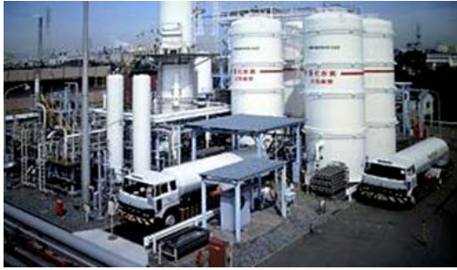
Photo 4: Vertical cylindrical tanks
