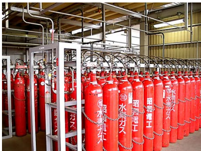
Photo 3: Filling compressed hydrogen in containers
