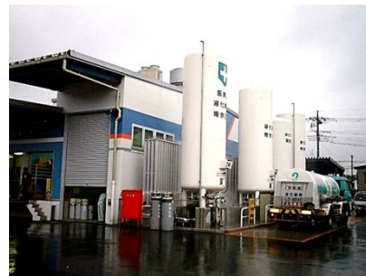
Photo 4: Storage and consumption of liquid oxygen
