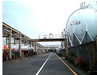
Photo 2: Storage and shipment of LPG
