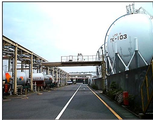
Photo 11: Designated Equipment (spherical reservoir)
