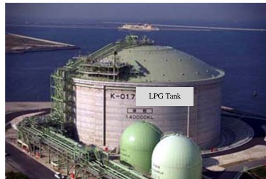
Photo 1: An example of low temperature storage tank
