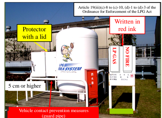
Photo 2: An example of bulk storage tank
